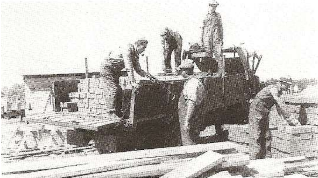
Loading a truck with material to complete an entire house.
