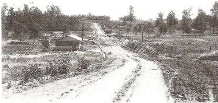
This is a road under construction on "D" Street with a bridge being built over the Palmetto Creek. The building is a canning plant which was called the "little" canning plant, as a larger plant was built on "E" Street.
